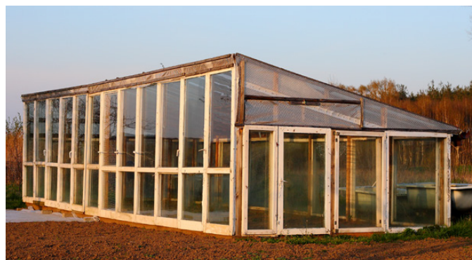
FIG. 3 Greenhouse built from recycled materials.
